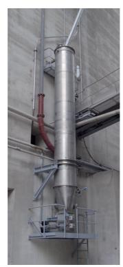
Partly visible cyclones for separation of the heated dust particles after the thermal treatment in the second preheater line
