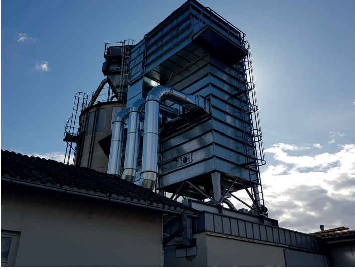
Economical solution: sepas extraction system for furniture production.
