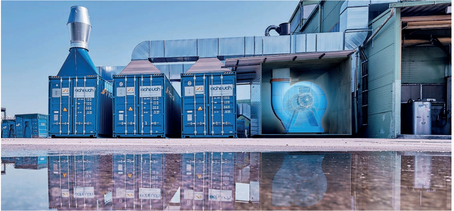
OEC odor filter at FCC Austria Abfall Service AG
