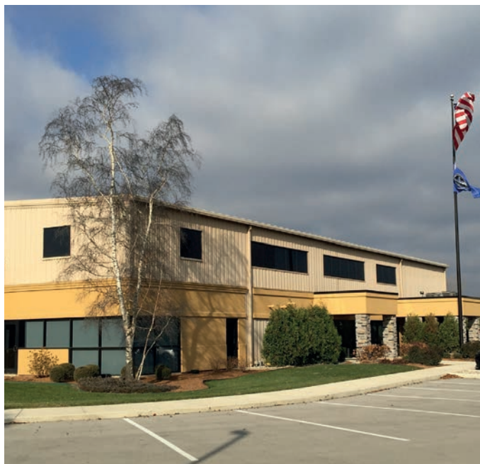
New Schust-Building, Auburn, Indiana.
