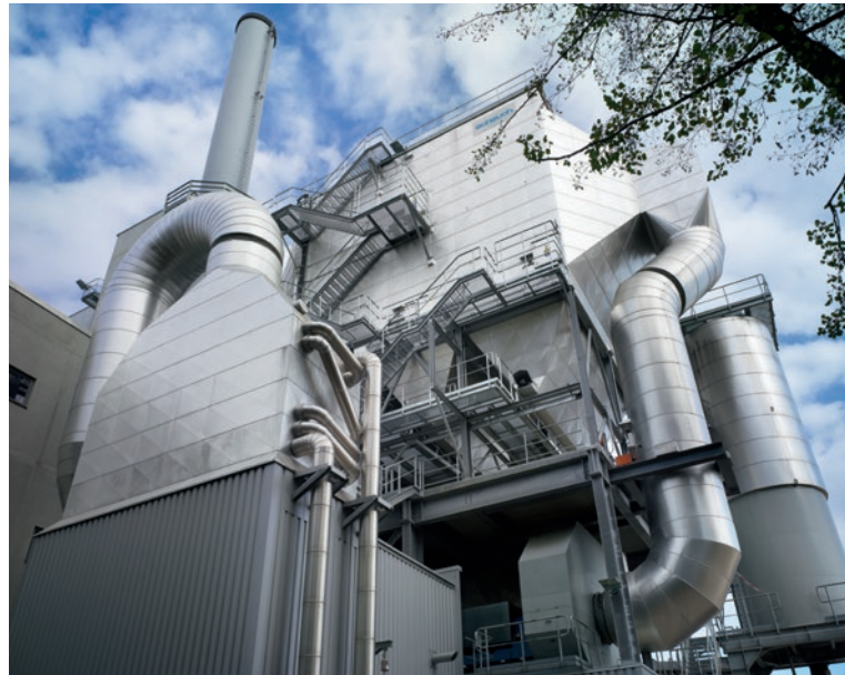
Useful heat for pellet dryers Project name: Unterbernbach Country: Germany Design: ercs – TYP 01 Boiler output: 43,7 MW thermal Fuel water content: w60
