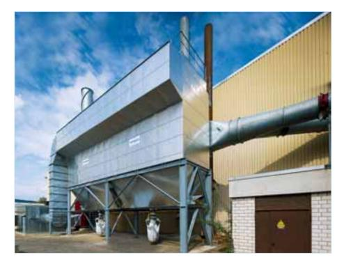
During the hot-dip galvanizing process, the flux material reacts with the molten zinc. According to TA Luft regulations, the gasiform (HCI) and dusty emissions (zinc chloride/ammonia chloride) created by this process must not exceed 20 and 5 mg/m<sup>3</sup>, respectively. In order to comply with these emission limits, a special collection, extraction and dedusting system is required, dimensioned in this case for 100,000 m<sup>3</sup>/h.
